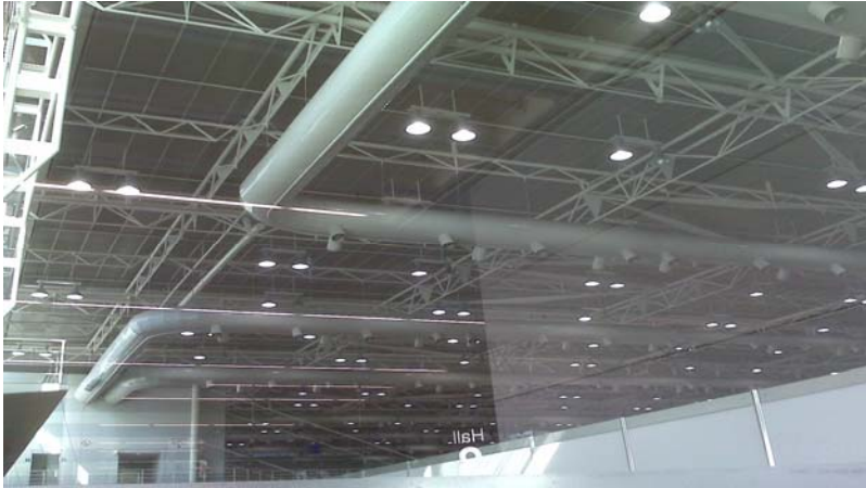
Figure 4 Sydney Convention & Exhibition Centre Ductwork Reticulation
