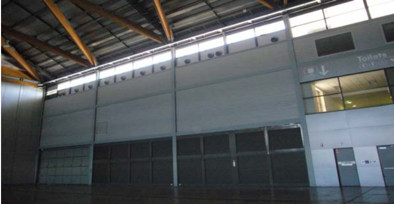
Figure 2 Existing Side Blow Diffusers
