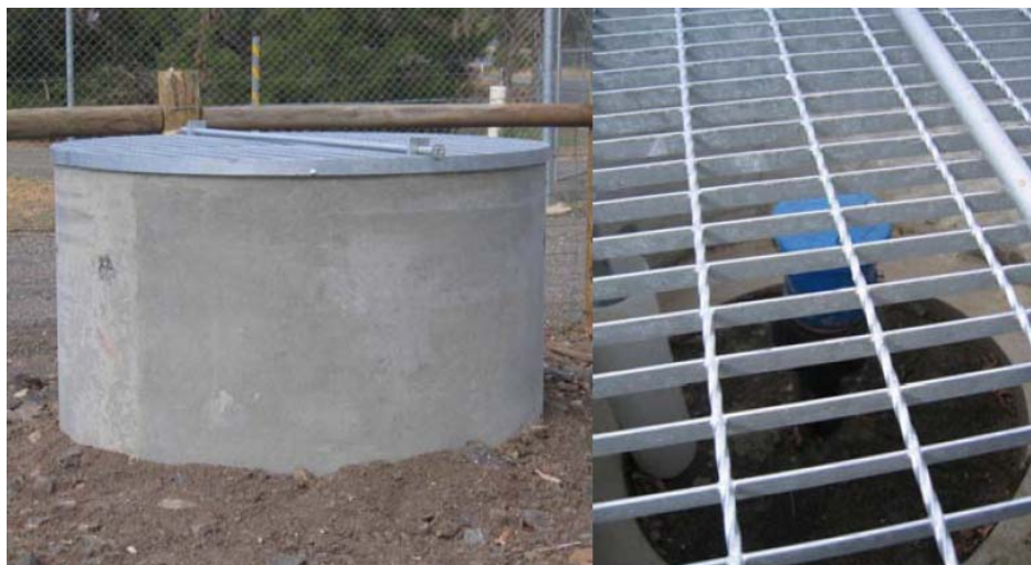
Figure 3.2 Example of a constructed air valve
