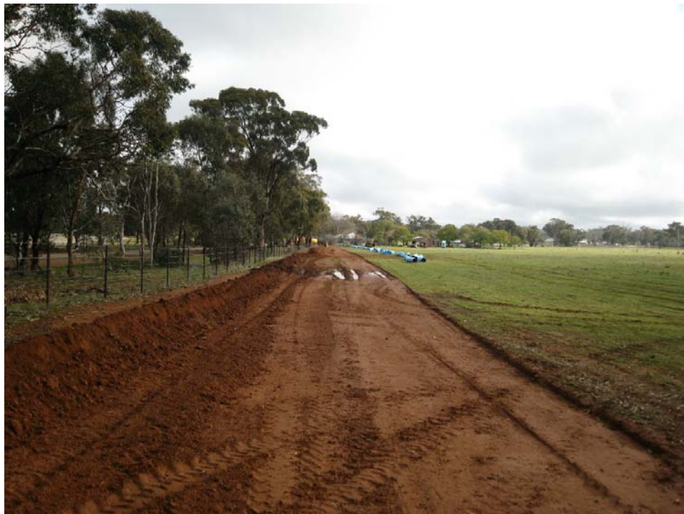
Figure 3.3 Prepared pipeline construction corridor
