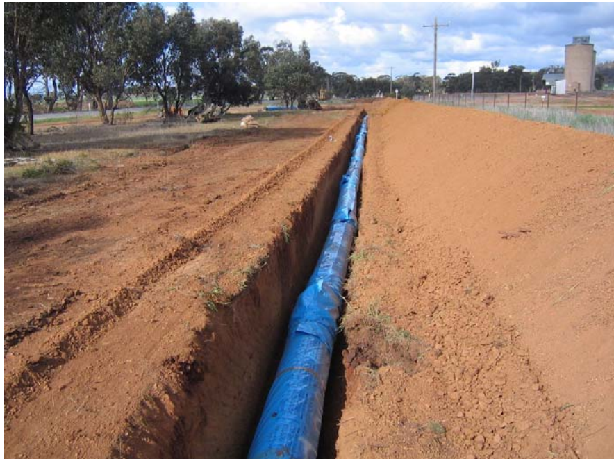
Figure 3.6 Covered pipe segments joined in the trench prior to replacement of excavated material
