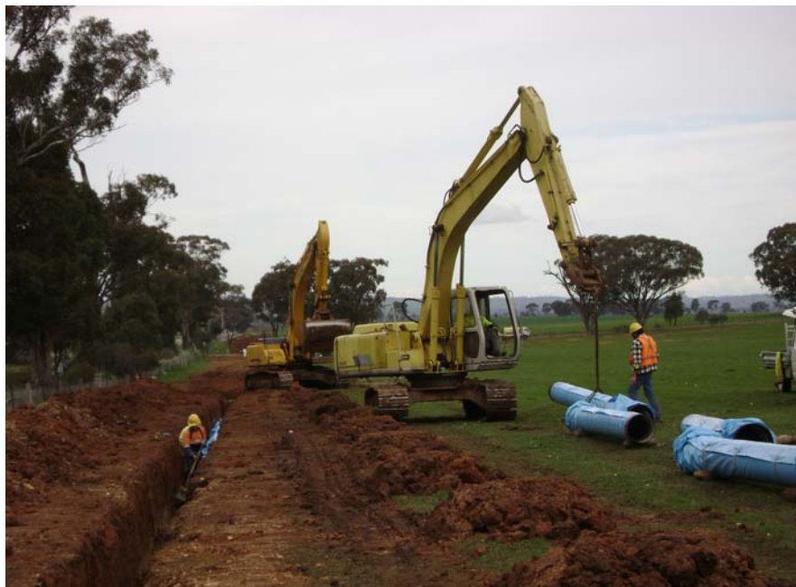
Figure 3.5 Lifting the pipe segments into the excavated trench (Stockinbingal to Temora pipeline)
