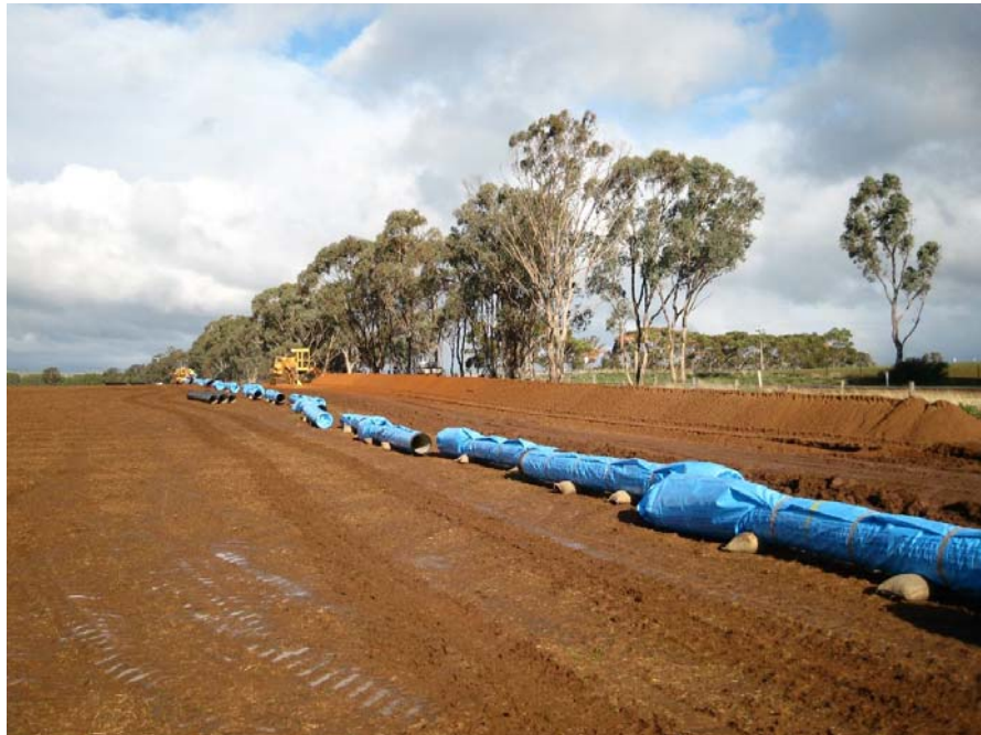
Figure 3.4 Stringing pipes along an excavated trench (Stockinbingal to Temora pipeline).
