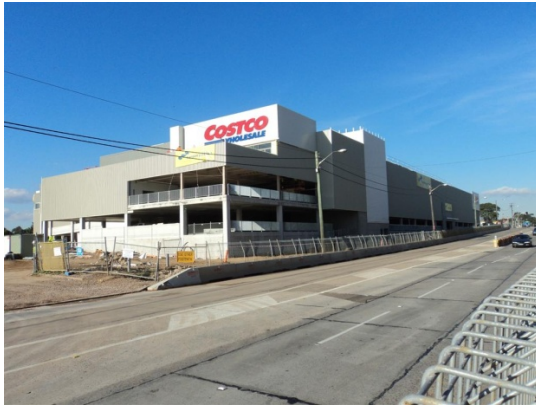
Figure 1 – View of site from Parramatta Road
