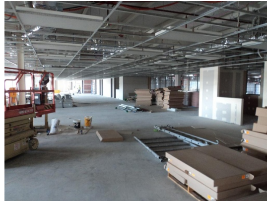
Figure 2 – View of Level 2 Office area presently under construction
