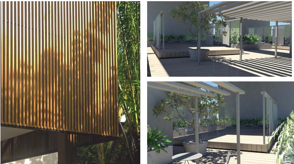
VERTICAL TIMBER BATTENS TO CENTRAL POD
