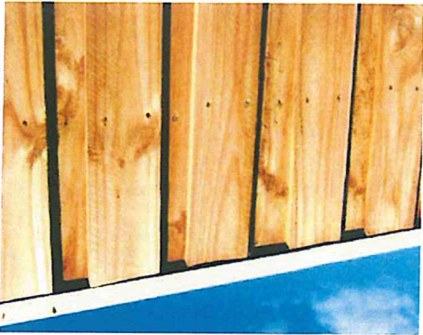
TIMBER PALING FENCE
