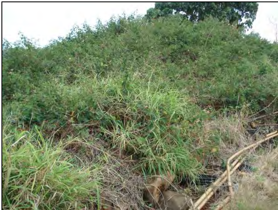
Figure 20: Substantial boulder wall (5m x 3m) overgrown with vegetation
