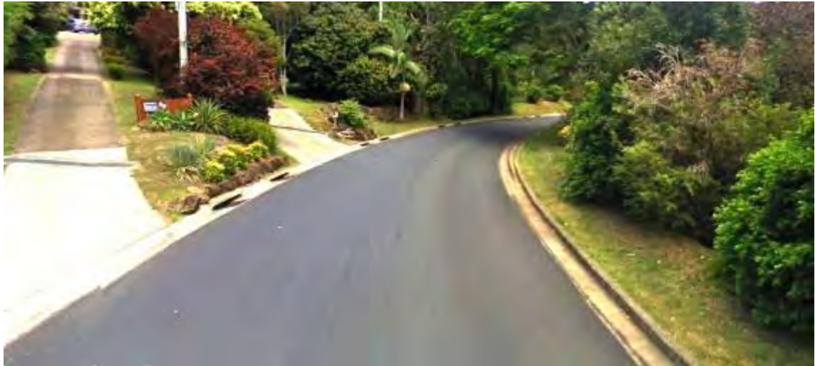
Figure 2.6: Parkes Lane – Existing Condition
