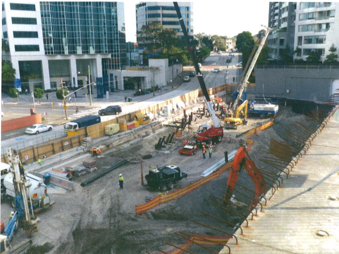
Figure 1 – Photo of site with works underway
