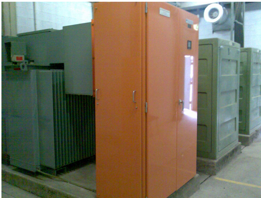
North Block Chamber Sub-station with Chamber and Pad Mounted Transformers
