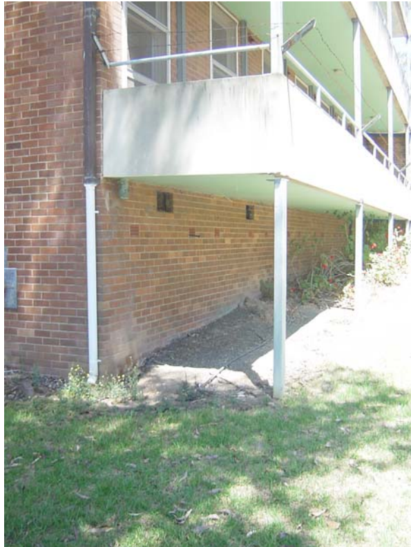
Northeast corner of existing East Block building showing evidence of settlement and possible salt crystallisation at foot of wall
