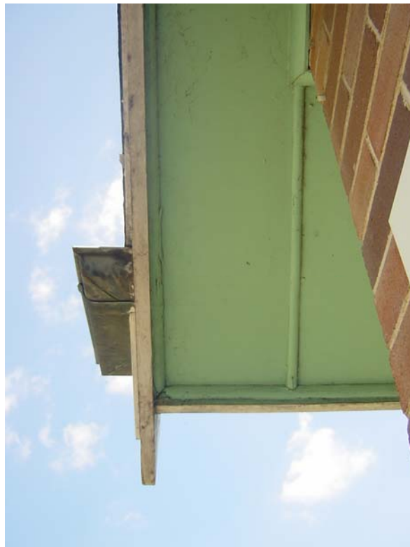
Possible cement bound asbestos eaves
