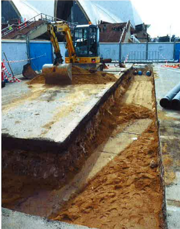
Figure 1 View looking north showing the exposed section of the c1860 sea wall located within a trench excavated for the installation of new services. (GML 2011)
