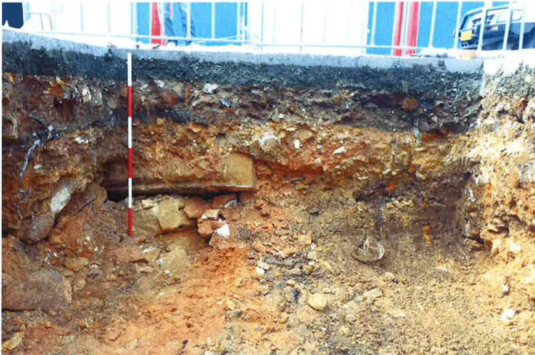
Figure 1 East section of the pit for the Gross Pollutant Trap showing fills associated with the construction of the Sydney Opera House. The pit was further excavated to a depth of over 2.5m resulting in the discovery of apportion of the oat slip. (Source: GML 2011)
