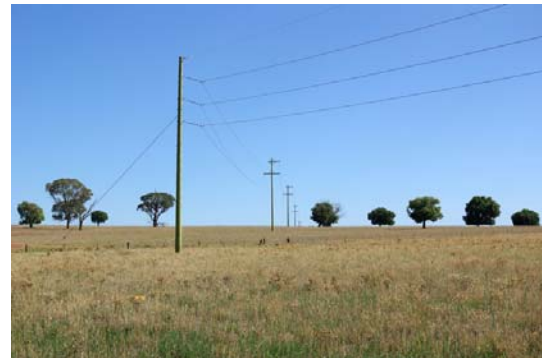
Plate 16. 132kV transmission line – typical angle pole.
