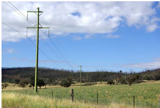
Plate 15. 132kV transmission line – typical intermediate pole.
