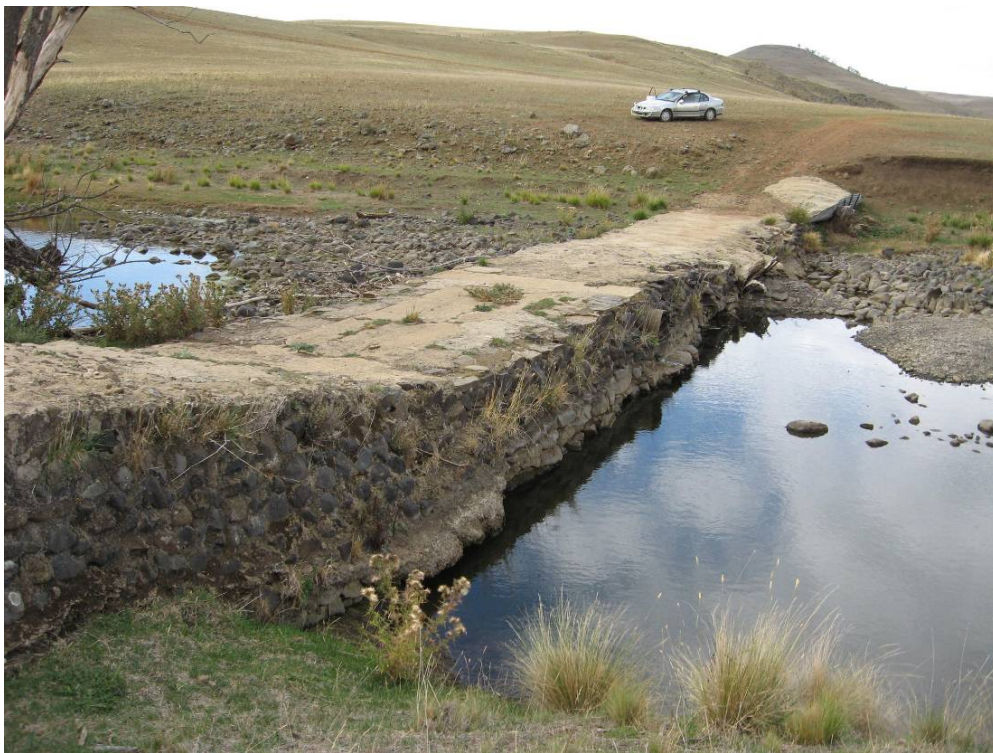
Plate 4 Causeway on Link Road looking east showing drop from outlet of culvert
