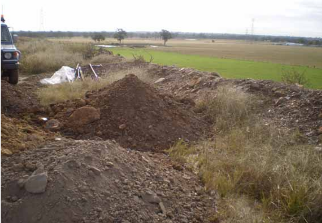
Photograph: 5 Test pitting on eastern bundwall, May 2010
