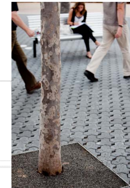
Permeable paving is proposed to collect stormwater. The hardscape collects and reuses stormwater on site for irrigation of the soft landscape.
