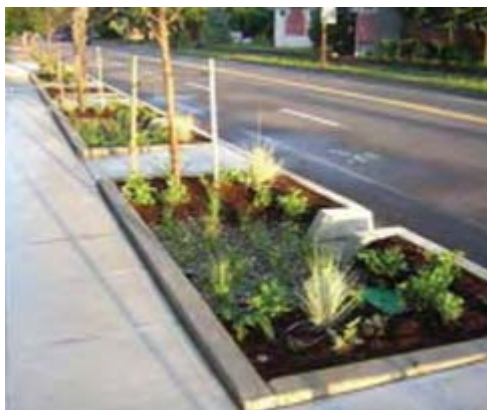
FIGURES 5.1, 5.2 AND 5.3 The WSUD measures proposed for the CODCD include the use of bio-swales within the site to slow stormwater and treat it prior to releasing it into stormwater systems, as well as the use of low-flow, WELs-rated tapware and ultra-low-flow urinals.
