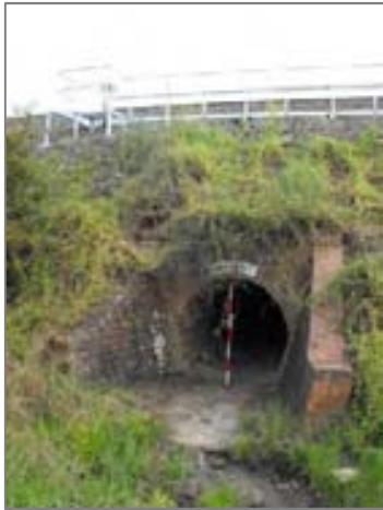
Down side of culvert 196.561 showing intact red brickwork of arch and brick floor (above and below).
