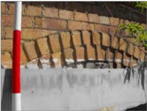
Up side of culvert 196.280 showing residual intact brickwork (above) and corrugated iron liner with concrete lintel with concrete infill (below).
