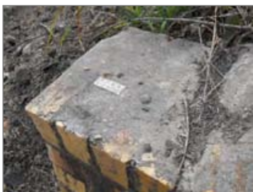
Survey mark on the upper surface of Up side wingwall.
