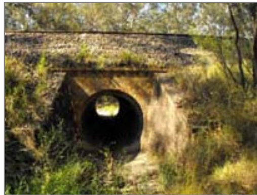
Downside of culvert showing intact brick arch with concrete pipe liner.
