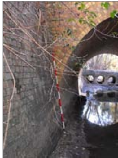
Down side view showing the country side, flat-angled wing walls and brick floor/apron. culvert.
