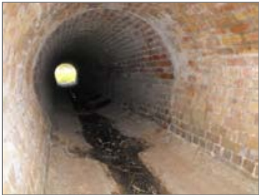
Up side of culvert 196.561 showing yellow brickwork of extension structure c1915-16 (above). The interface of the extension to the original c 1860 brick arch structure can be clearly seen (below).
