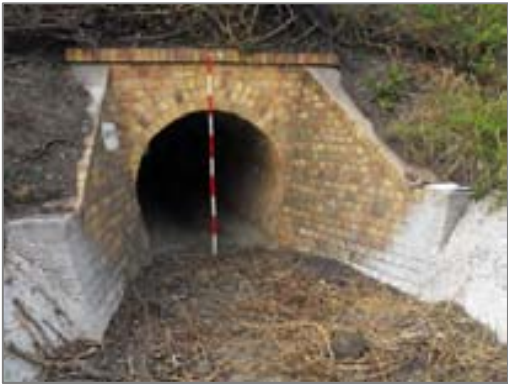
Up side of culvert 196.561 showing yellow brickwork of extension structure c1915-16 (above). The interface of the extension to the original c 1860 brick arch structure can be clearly seen (below).
