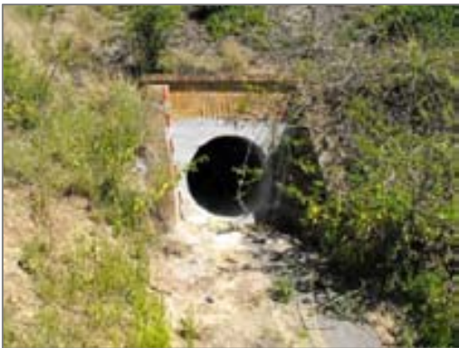
Up side of culvert 196.280 showing residual intact brickwork (above) and corrugated iron liner with concrete lintel with concrete infill (below).
