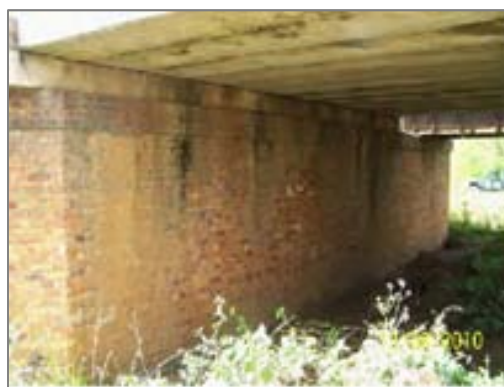
Metal beams had been replaced by precast concrete sections.
