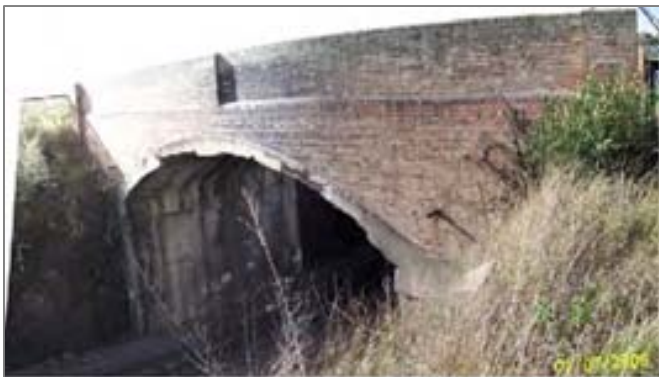
Two views of the westerly side of the Old North Road Overbridge at Allandale, noting in particular the deteriorated condition of concrete work.
