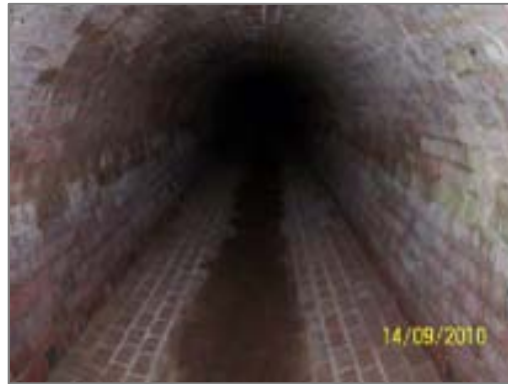
Internal view of culvert showing intact dish brick floor.
