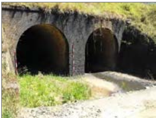
Northern elevation showing face of brick extension c1915-1916.
