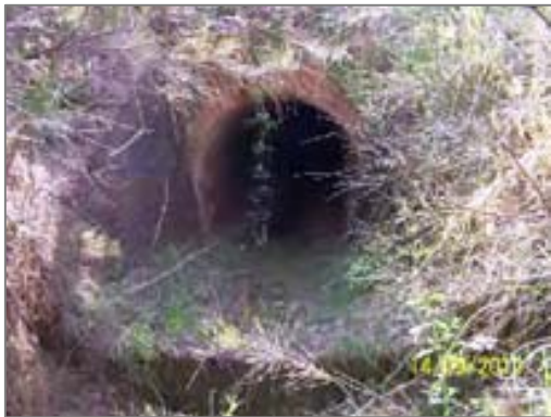
Downside intact brick arch culvert with brick floor and external dish drain.
