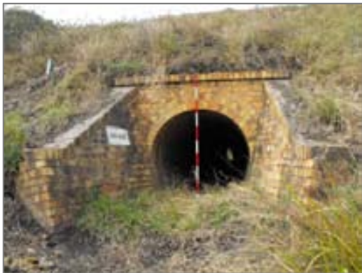
Upside of culvert 196.481 showing intact brick arch and brick floor.
