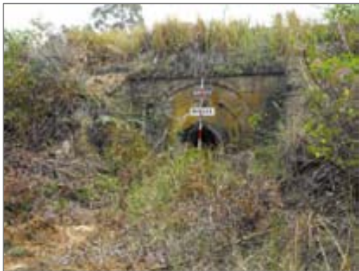
Downside of culvert 196.481 showing very early concrete pipe insert and concrete infill.
