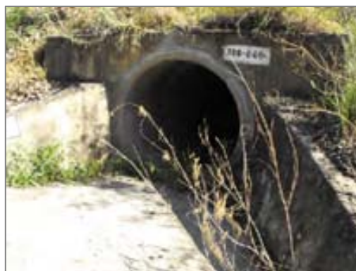
Upside view of concrete pipe culvert extension and cast in place concrete wing walls.
