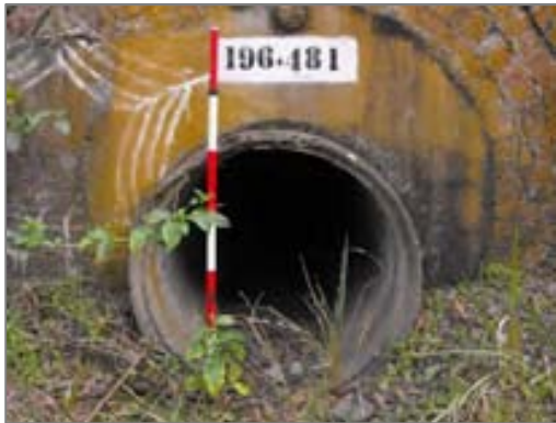
Downside of culvert 196.481 showing very early concrete pipe insert and concrete infill.
