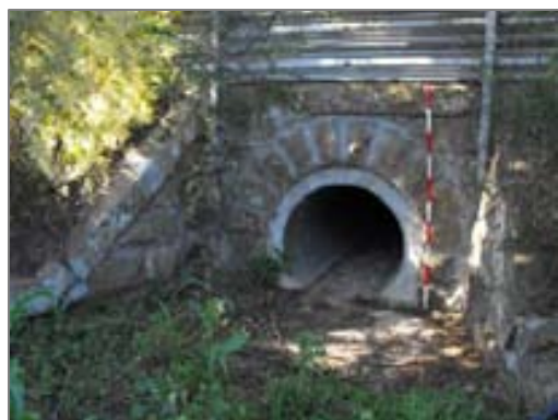
View of downside stone culvert showing concrete sleeve insert.
