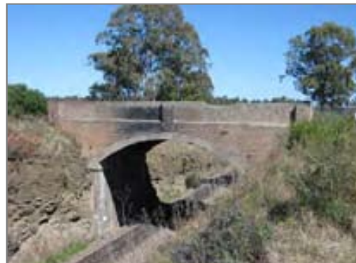
Two views of the westerly side of the Old North Road Overbridge at Allandale, noting in particular the deteriorated condition of concrete work.
