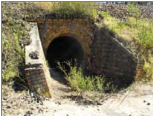
Upside of culvert showing intact brick arch with concrete pipe liner.
