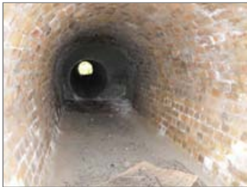
Upside of culvert 196.481 showing intact brick arch and brick floor.
