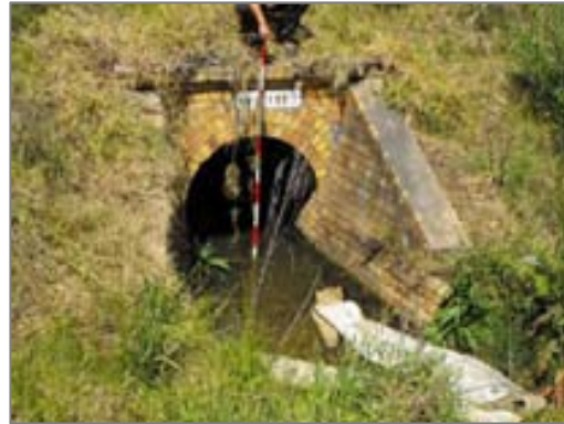
Up side of culvert 195.133 showing the elevated rail corridor (left) and unmodified brick arch of the 1915-16 extension (above).
