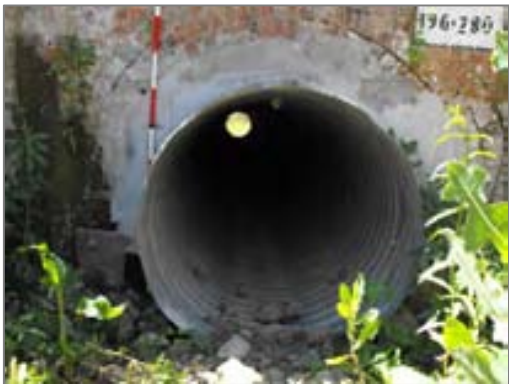
Downside of culvert 196.280 showing intact brickwork (above) and corrugated iron liner with concrete infill (below).
