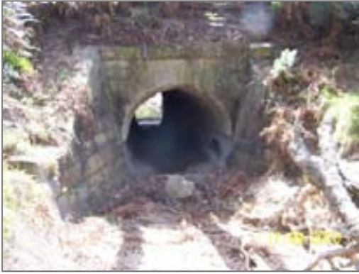
Wide view of the Down side elevation of the stone culvert (left) and detailed view of headwall, portal and insert (right).
