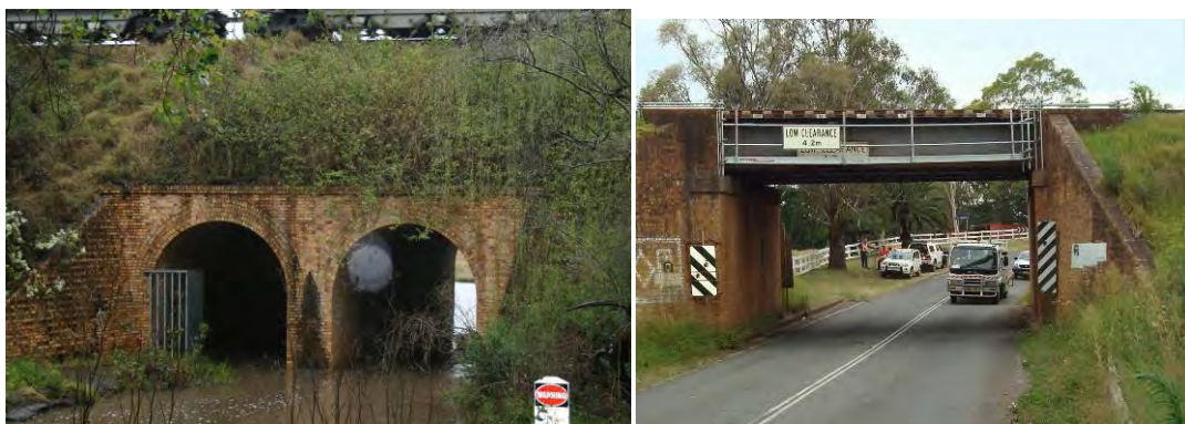
Figure 7.20 Existing Stony Creek Brick Arch Culverts (Left) and Existing Wollombi Road Underbridge (Right)
