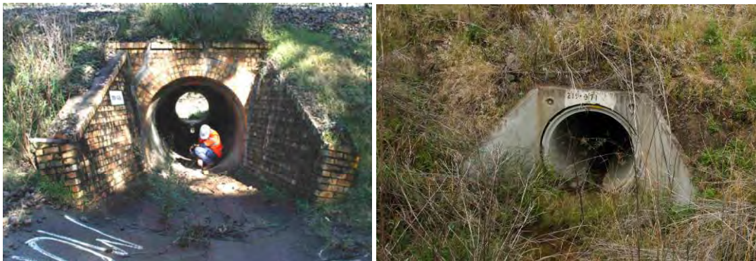
Figure 7.14 Typical Cross Drainage Structures
