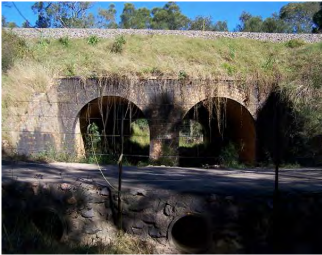
Figure 7.26 Existing Unnamed Tributary of Anvil Creek Brick Arch Culverts (chainage 207.776 kilometres)
