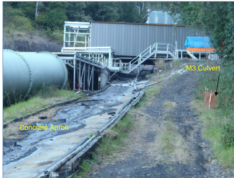
Photo 1: Concrete Apron, Removed Conveyor Alignment and the Junction of the Culvert (M3 Culvert) with this Alignment
