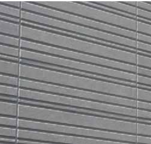
Photo 6.2.27 Hebel wall with horizontal pattern
