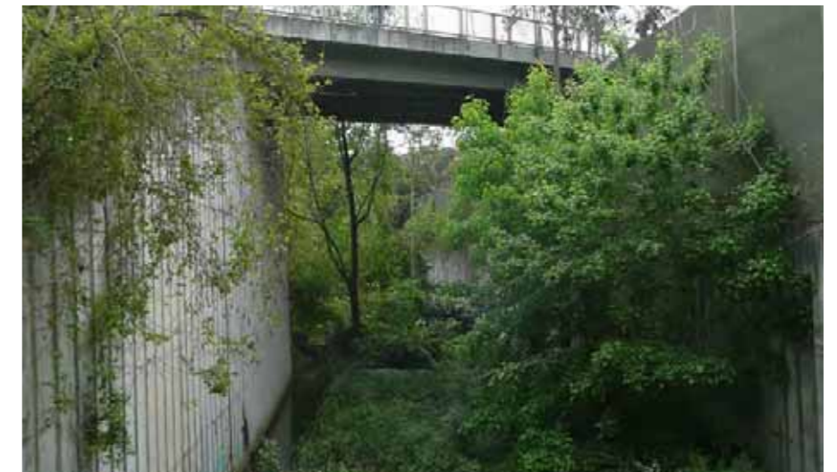
Photo 3.31 View of drainage line under Kirkham Road Bridge.
