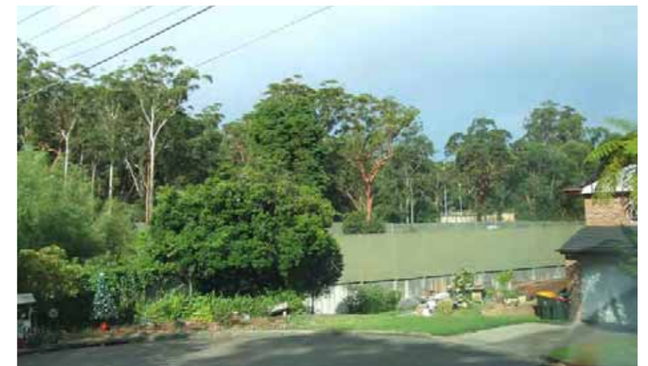
Photo 3.32 View from Meadow Close off Devlin Crescent, Channel Wall and M2 noise wall.
