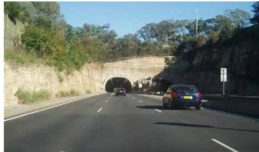
Photo 3.35 View of eastern tunnel approach.
