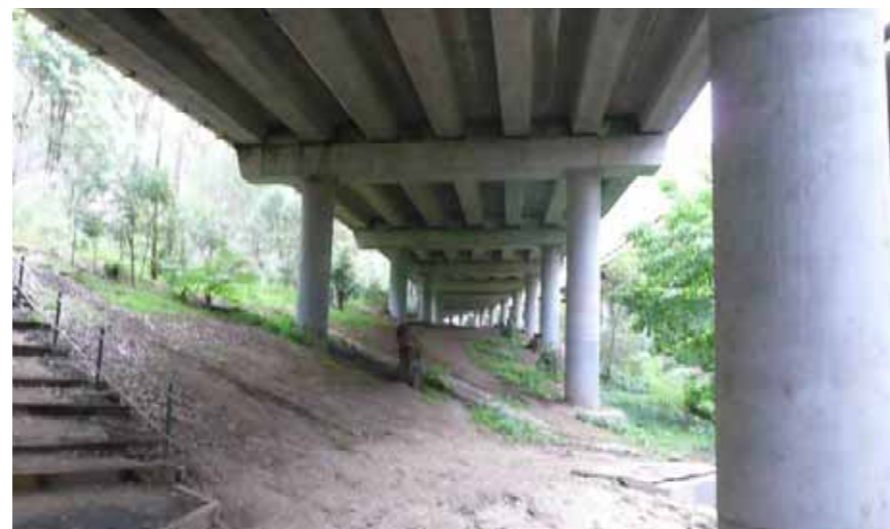
Photo 3.29 View of space under existing westbound bridge over Devlins Creek.
