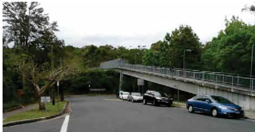
Photo 3.33 View of Kent Street pedestrian bridge and noise wall.
