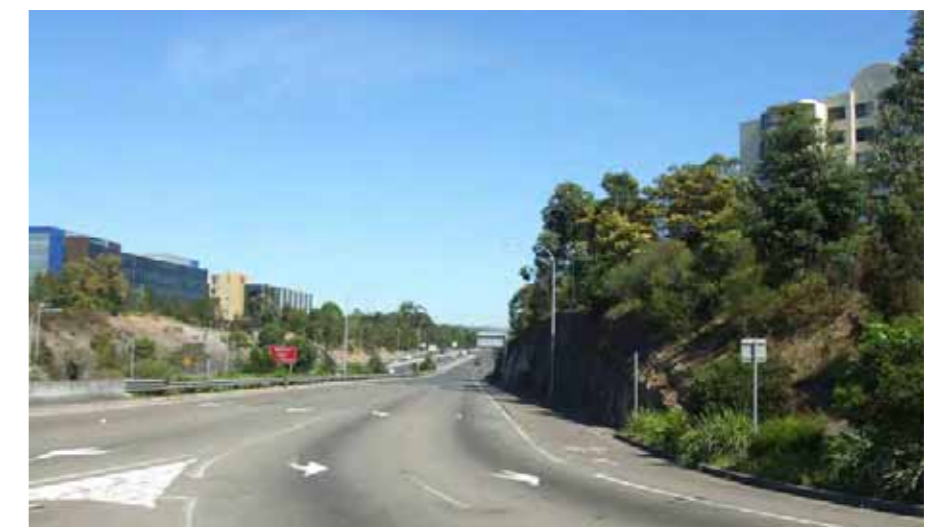
Photo 3.44 View from Lane Cove Road of office/commercial buildings overlooking the motorway.
