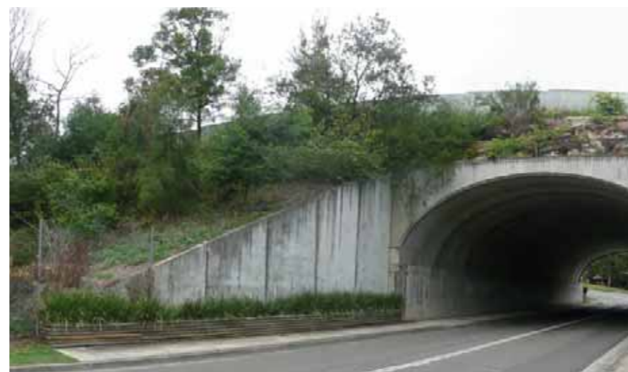
Photo 3.41 View of Busaco Road headwall, illustrating sandstone headwall, to be replaced by vertical headwall and noise wall on top.
