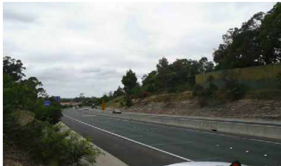
Photo 3.46 View of cutting opposite Vimiera Road transmission tower looking east.
