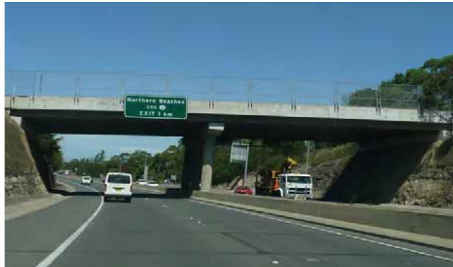
Photo 3.45 View of Christie Road Bridge and abutments.
