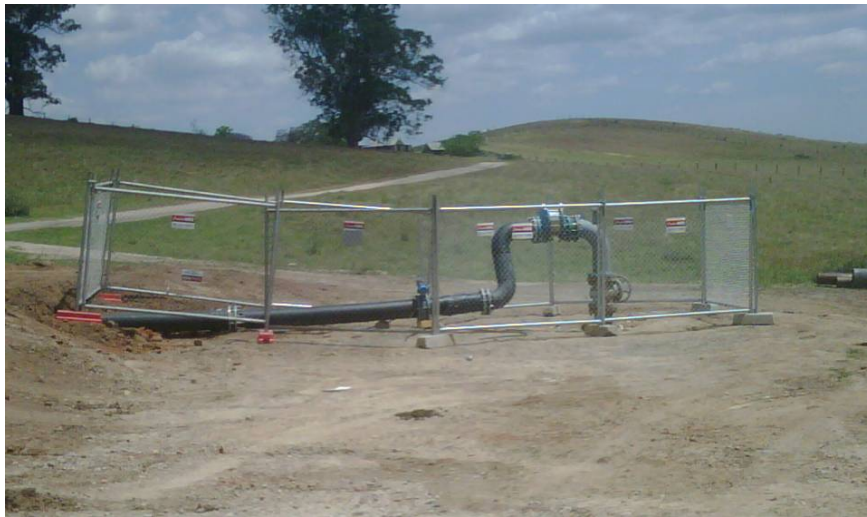
Figure 6 – Wellhead Installation
