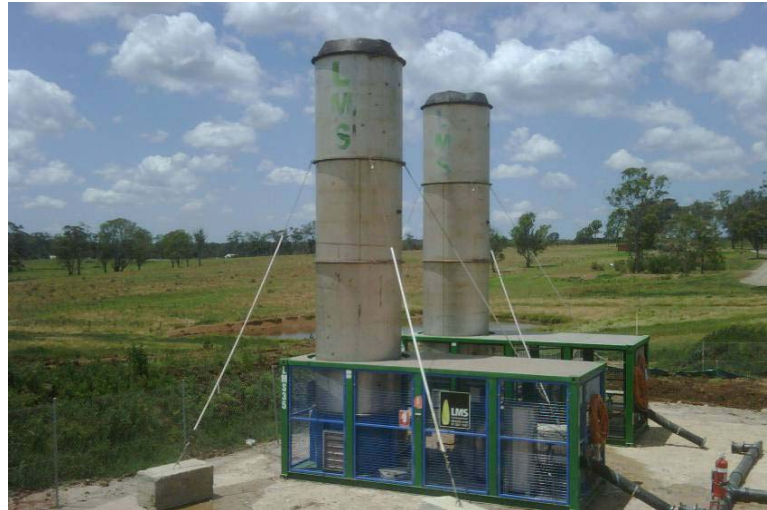
Figure 9 – Enclosed Goaf Gas Flaring Units
