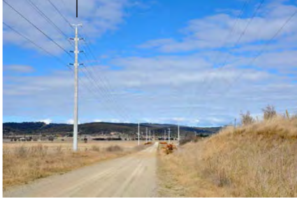
Double circuit 132kV powerline (supporting structure) along road
