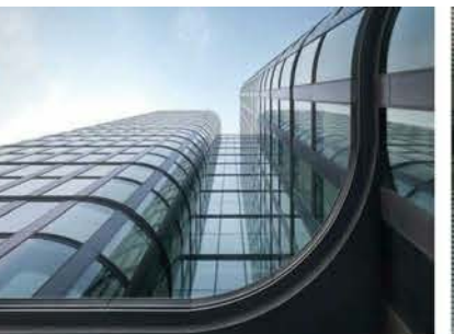
6. Curved, doubled glazing curtain wall
