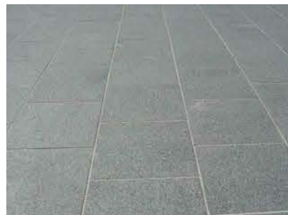
1. Stone cladding - Austral black, honed face
