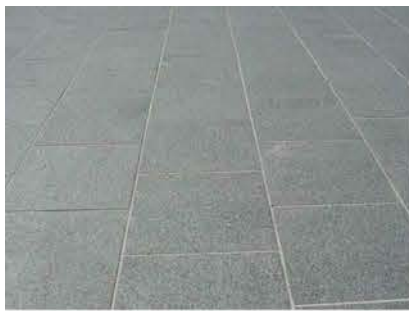
1. Stone cladding - Austral black, honed face
