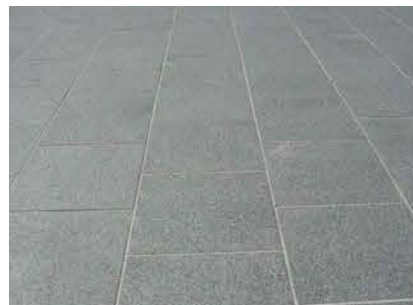
1. Stone cladding - Austral black, honed face
