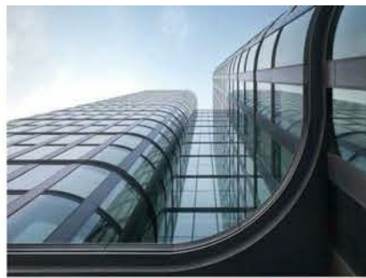
6. Curved, doubled glazing curtain wall
