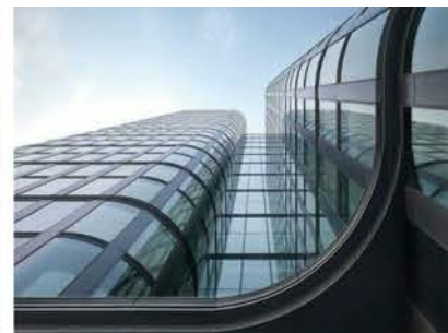
6. Curved, doubled glazing curtain wall
