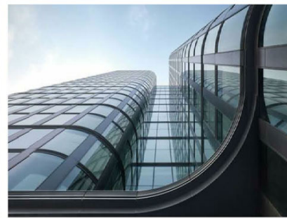
6. Curved, doubled glazing curtain wall
