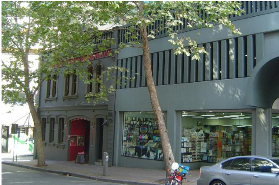
Figure 11: Former North Sydney Fire Station, View from north on Walker Street
