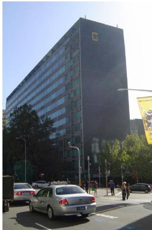
Figure 16: The MLC Centre, View from south west
