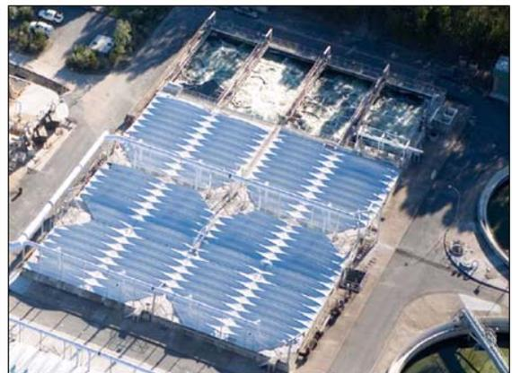
**Figure D-8 FRP Arc Span Anaerobic and Anoxic Zone Covers**
