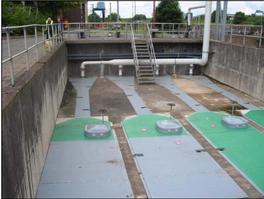
**Figure D-4 Flat Trafficable FRP Inlet works Covers**
