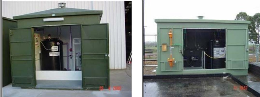
**Figure 3-2 Example Self Contained Chemical Dosing Unit**
