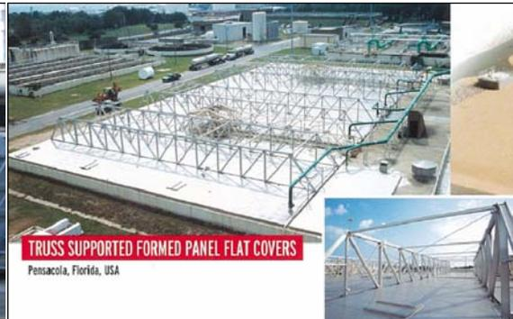
**Figure D-7 Fixed Aluminium Flat Cover Arrangements**
