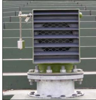
**Figure D-5 Weighted Air Inlet Dampers**
