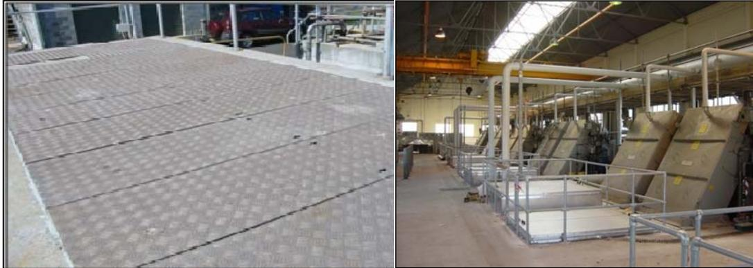
**Figure D-2 Example Aluminium Inlet Works Covers**
