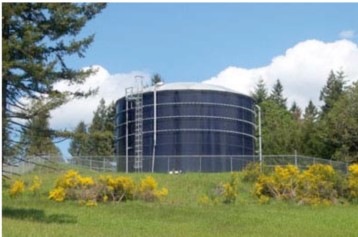
Figure 5.13 A typical recycled water reservoir (10m diameter)
