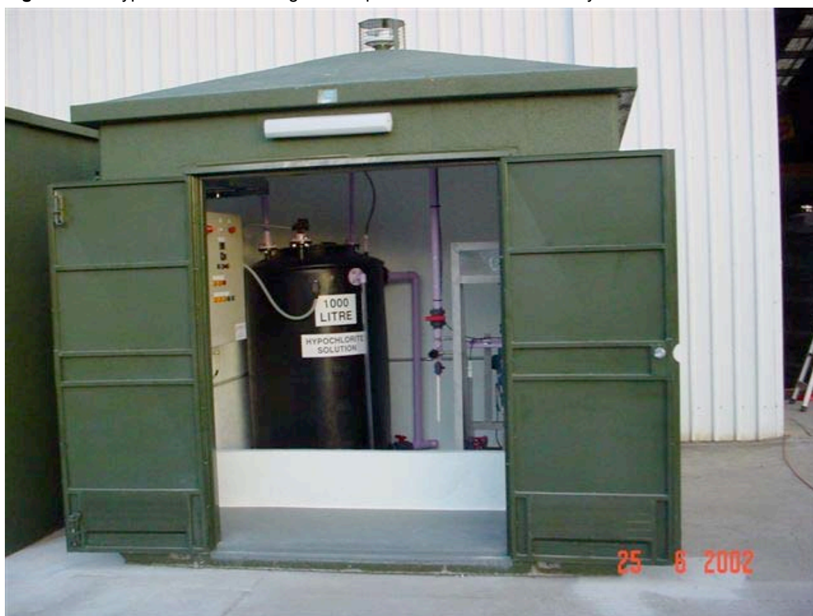
Figure 5.10 Typical chlorine dosing unit for potable water distribution systems
