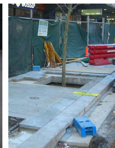
Construction of a planter tree in Sydney (Kings Cross)
