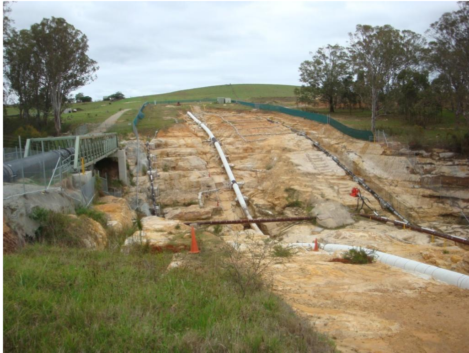
Figure 46: Decoupling of Pressurised Gas Pipelines and Water Main from Ground Movements, Mallaty Creek
