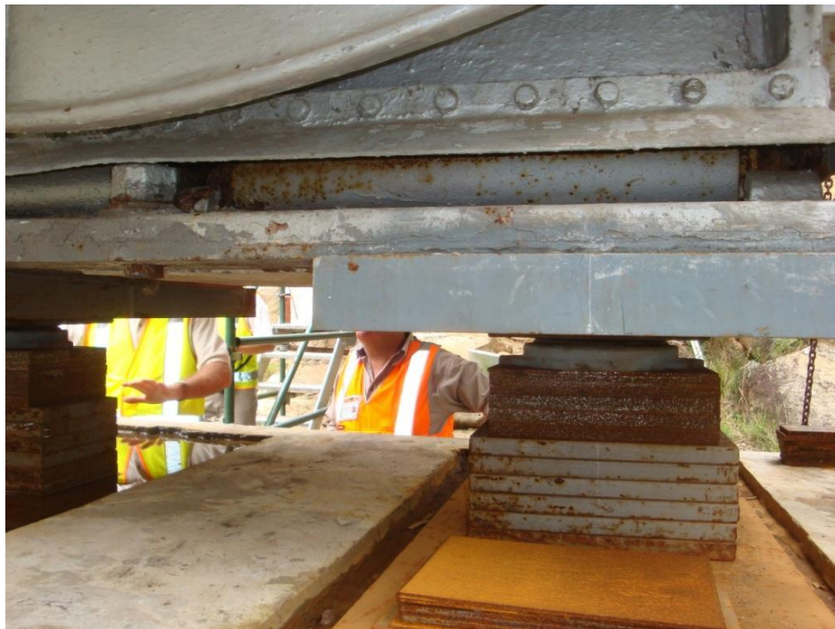
Figure 45: Jacking and Packing of Simpsons Creek Aqueduct to Accommodate Upsidence
