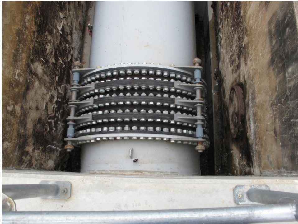
Figure 44: Rubber Bellows Fitted into Simpsons Creek Aqueduct to Mitigate Valley Closure
