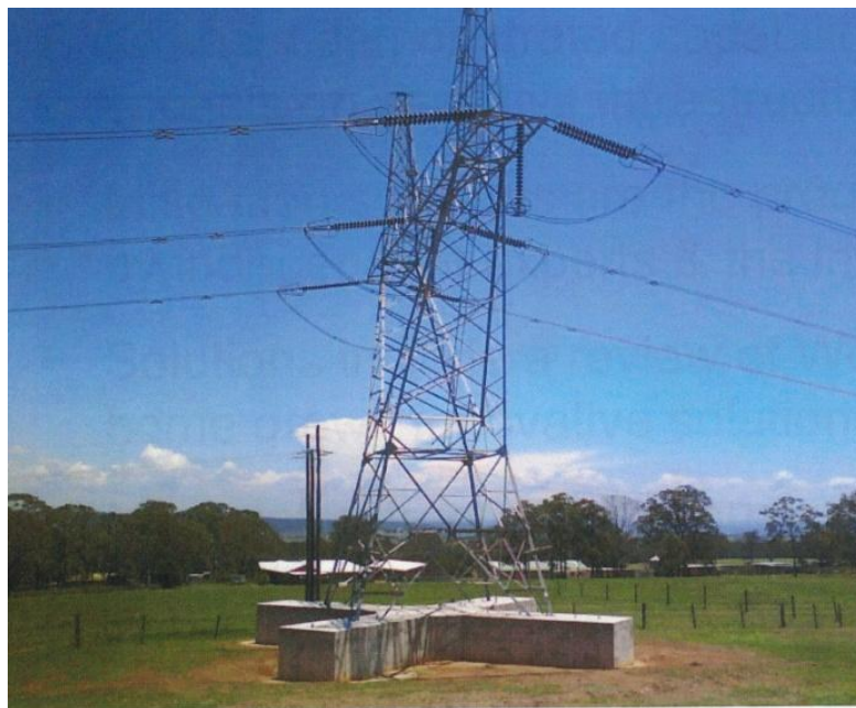
Figure 47: A High Voltage Transmission Tower above West Cliff Colliery Retrofitted with a Rigid Cruciform Foundation to Mitigate Differential Subsidence Movements 454
