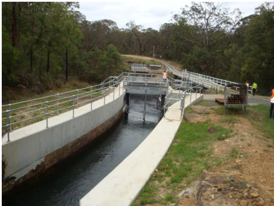
Figure 43: Increase in Height of Walls of Upper Canal to Mitigate Vertical Displacement
