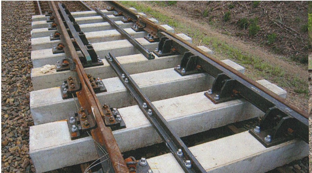
Figure 48: Switch Points and Real Time Monitoring Installed in the Main Southern Rail Line above Longwall 703 at Appin Colliery to Manage Mining Induced Strain in the Rails 455
