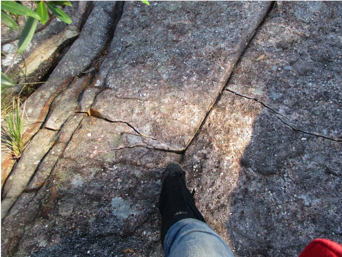
Plate 18: Eastern Tributary, MRIP08, Photo Point 8, cracking – autumn 2020.
