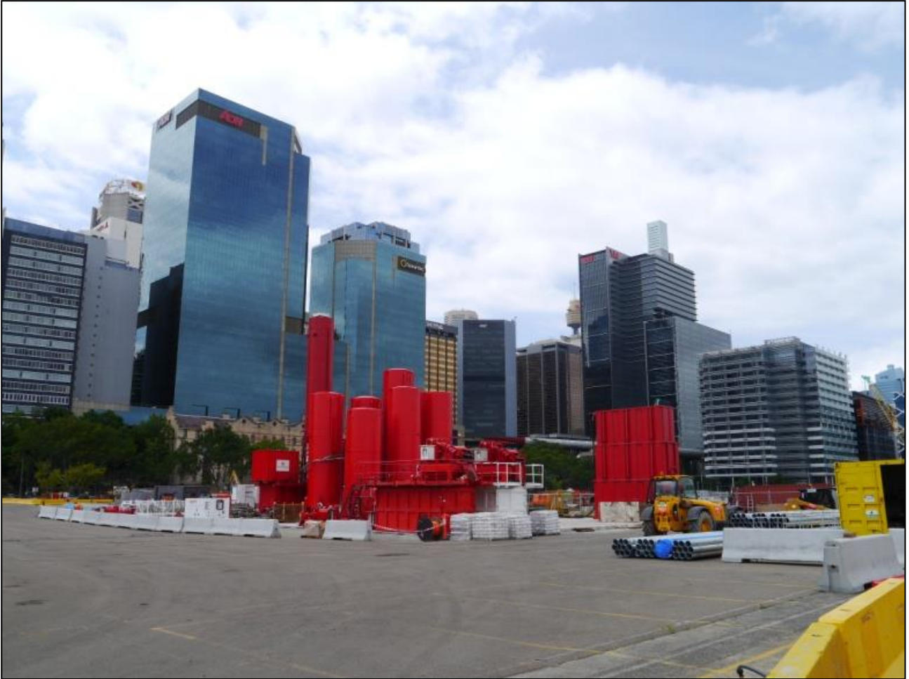
Plate 6: Typical silo, batch plant and de-sander set-up (Photograph courtesy of Menard Oceania)
