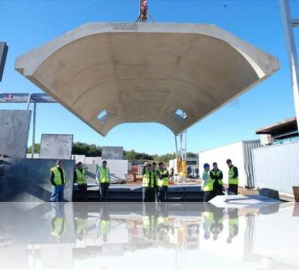
Precast vaulted slab (optional chilled beam/slab system)
