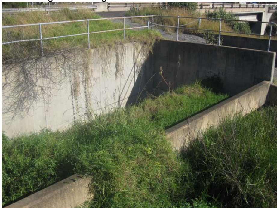
Figure 7: Overgrown Sediment Basin in Area 6.
