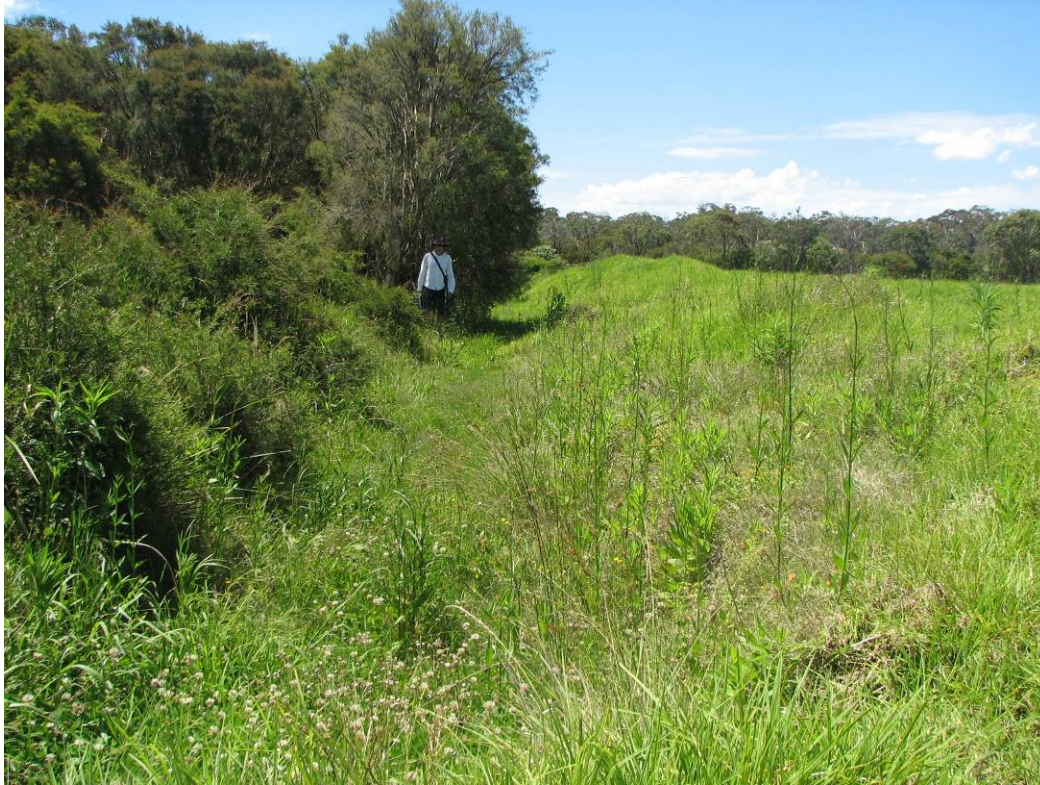
Figure 19 Ditch draining the western perimeter of the site. This ditch drains the area adjacent to the bund and maintains sufficient dryness in the site hydrology to allow the persistence of the adjacent swamp forests immediately to the left.
