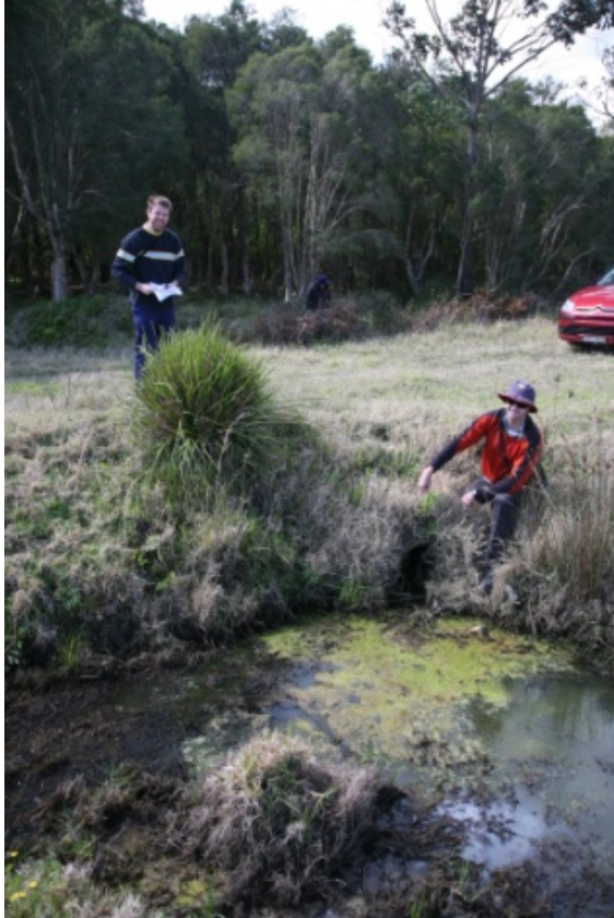
Figure 3 Culvert near north western corner of site that collects runoff from site drainage ditches and directs flow under the road reserve. Note the dominance of pasture grasses on the banks and growing into the ditch.
