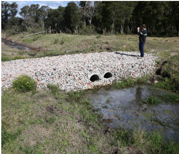
Figure 7 Informal crossing in electricity easement looking downstream towards the Freshwater Wetlands EEC. Note that grasses in the channel upstream of the culverts are green, whereas grasses downstream of the culverts are brown where they may have been killed by salt water intrusion. The obstruction across the easement created by the culverts probably limits the extent of saltwater intrusion.
