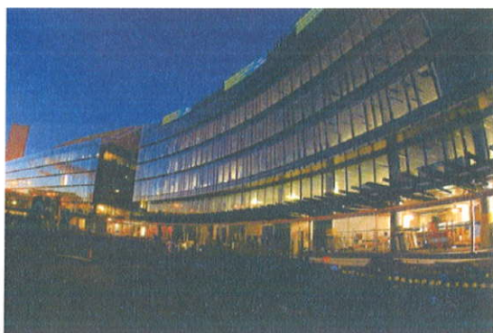
Figure 5: Current western façade
