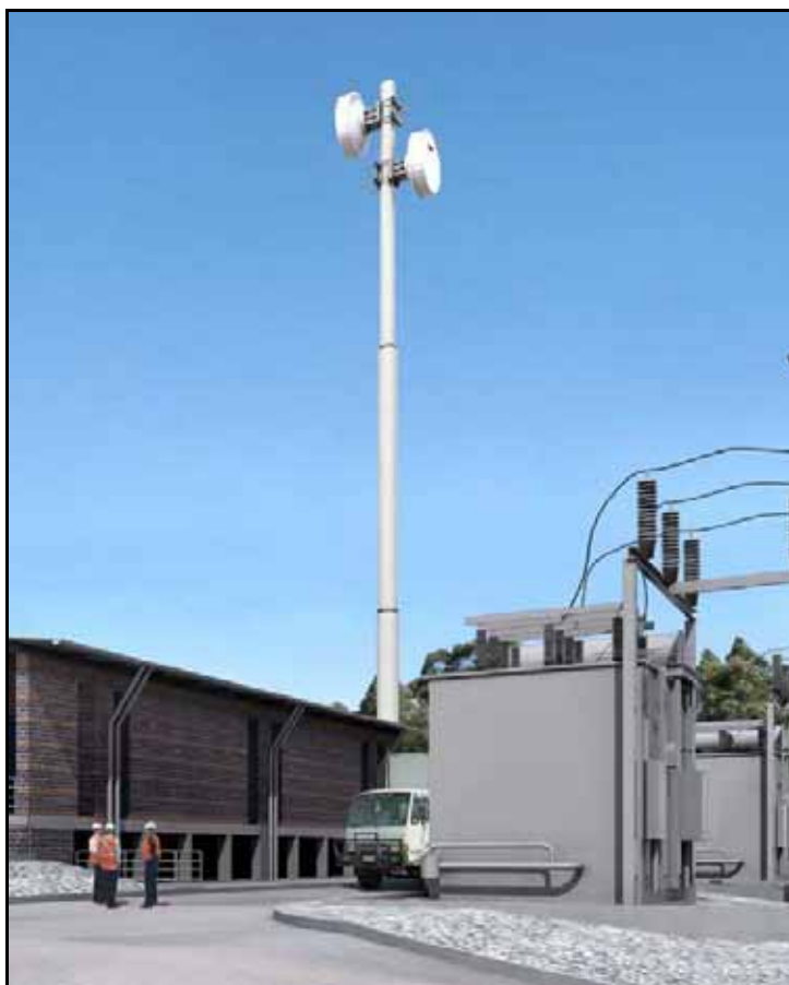
Figure 10.2 Example of slimline communications pole with dish antenna
