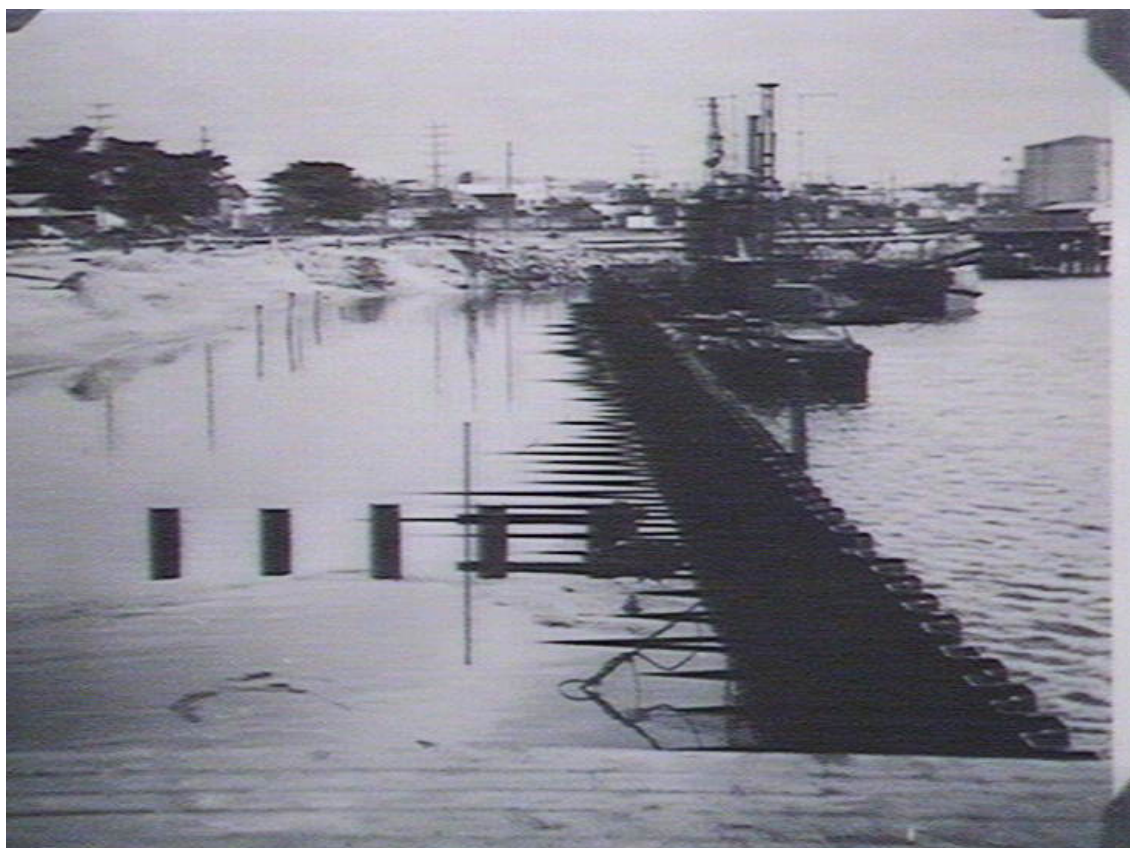
Figure 2.5 c1910 photograph showing the retaining wall in place for the construction of Lee Wharf. Note the sandy ground to the left of the image. This represents the northern edge of the original Honeysuckle area. (Source: GPO 1 — 20660)
