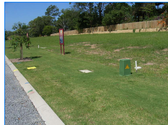
PHOTO 6 - EXAMPLE OF SERVICES WITHIN NATURE STRIP.
