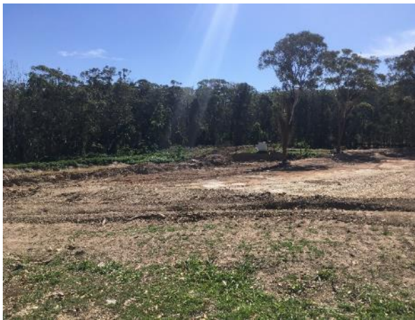
Plate 2.1 View west showing clearing for effluent ponds/water storage dam and associated vegetation removal
