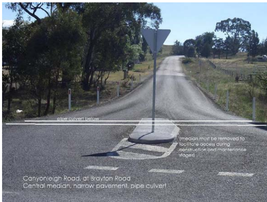
Figure 2-2 Brayton and Canyonleigh Roads intersection
