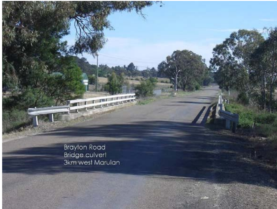
Figure 2-1 Brayton Road narrowing over bridge culvert
