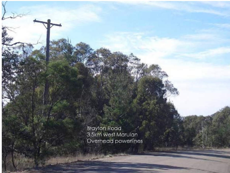
Figure 2-3 Brayton Road overhead powerlines
