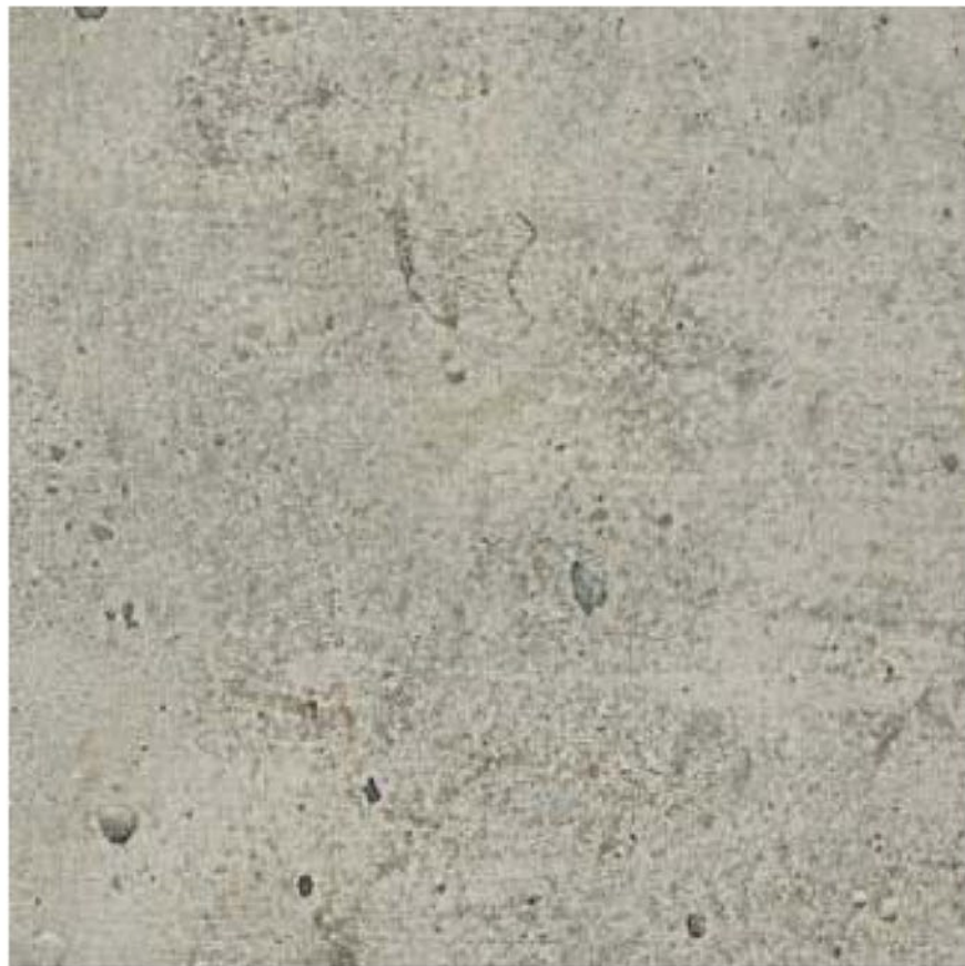
USBS - CE: 01 - Concrete floors
