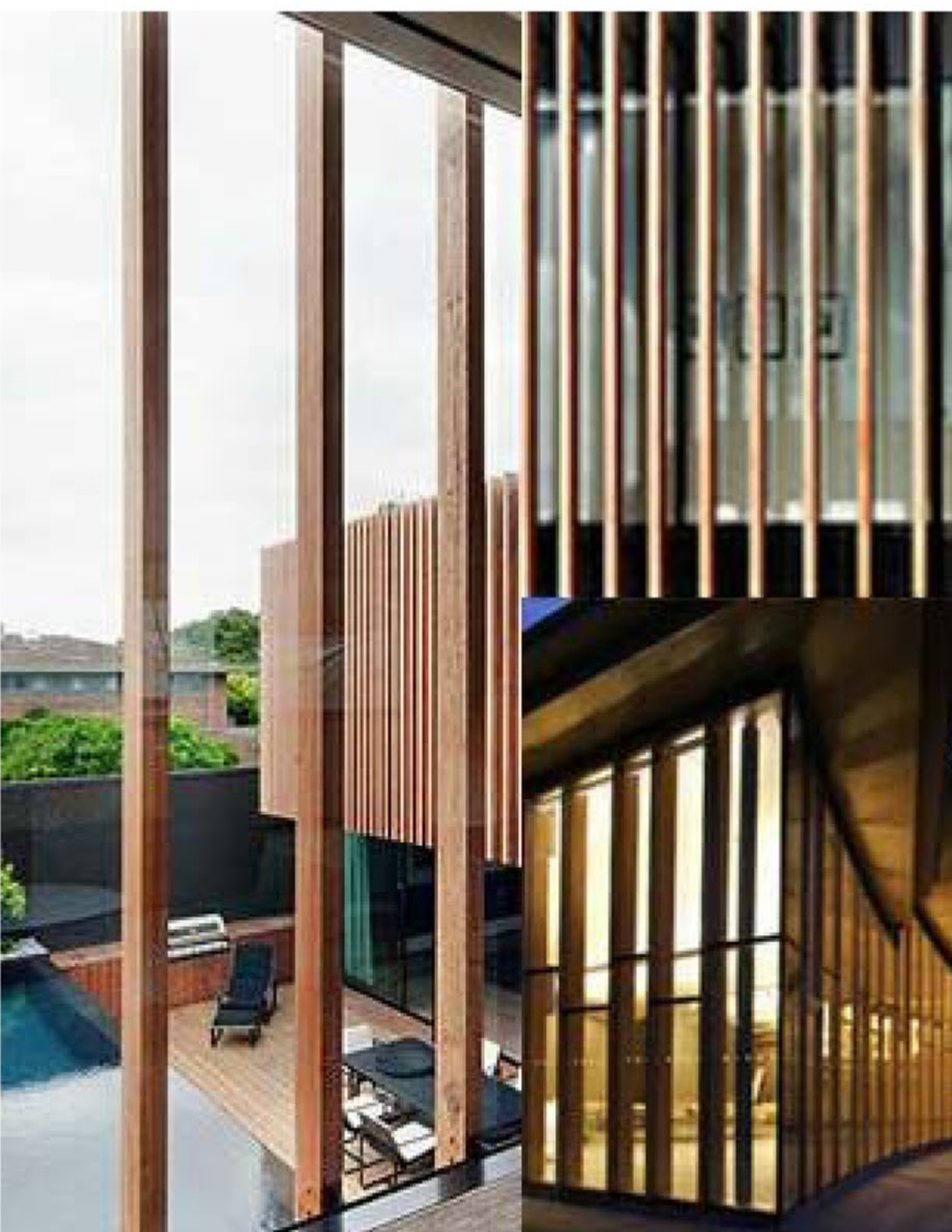
USBS - CL: 01 - Glass and timber glazing
