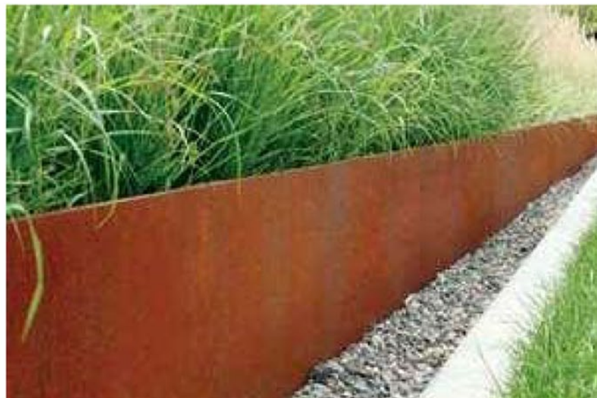
USBS - CD: 01 - Corten Steel retaining walls
