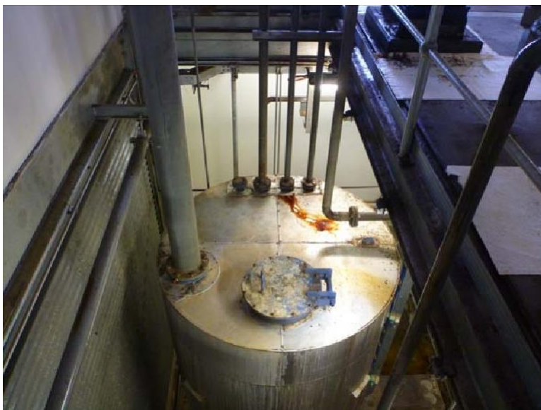
Figure 22 Tank vent collection system
