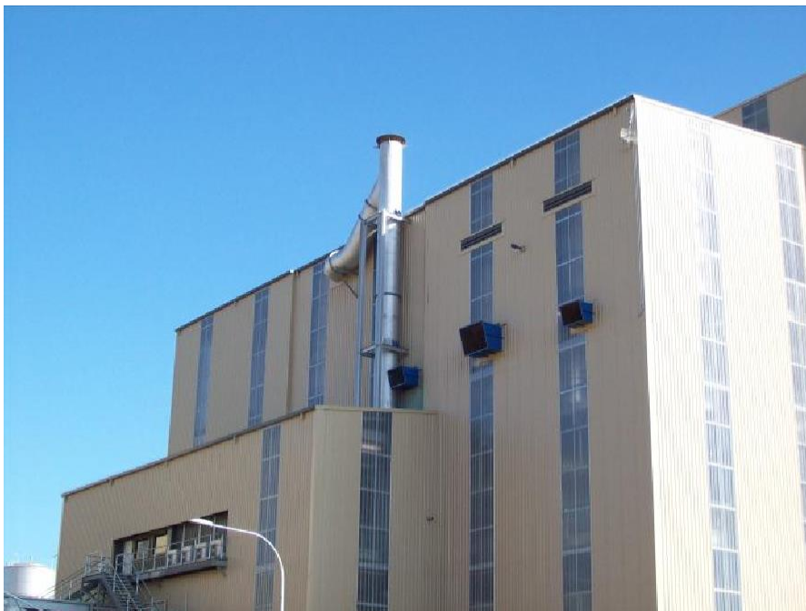
Figure 9 Seed Preparation Plant - Combined Vent
