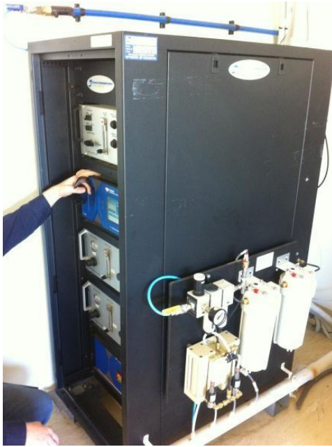
Figure 25 Continuous Emissions Monitoring System
