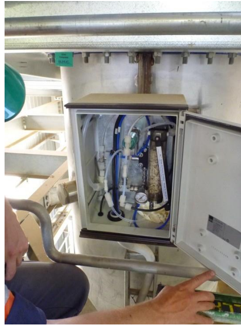
Figure 25 Continuous Emissions Monitoring System
