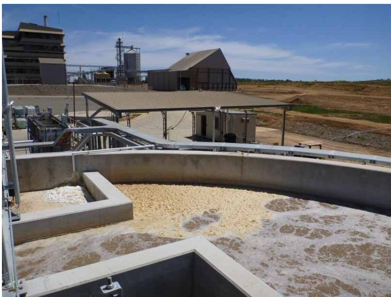
Figure 17 Aeration tank in the wastewater treatment plant
