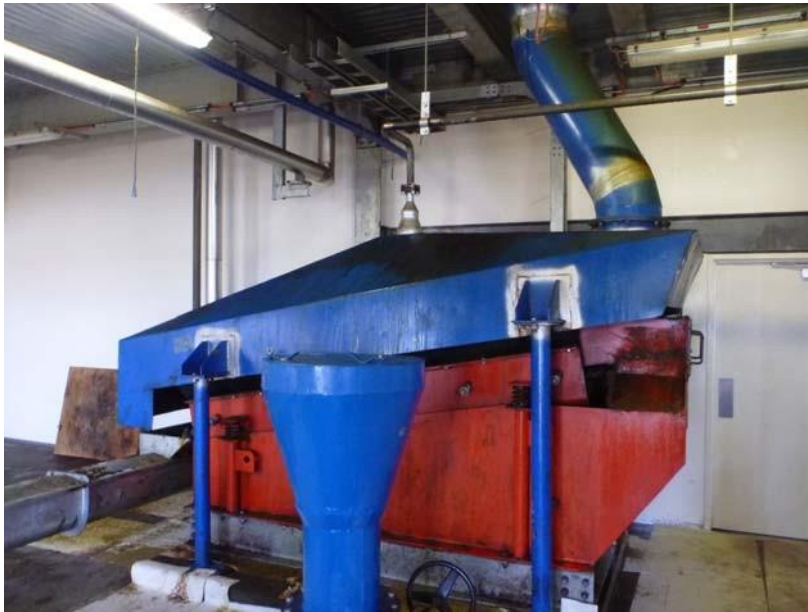
Figure 23 Oil screen with air collection hood and extraction system
