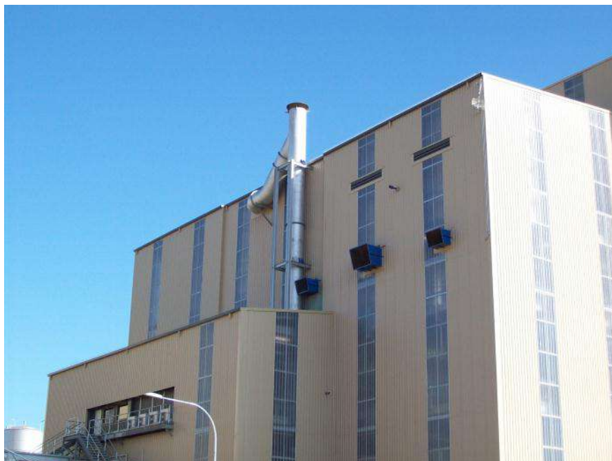
Figure 13 Seed Preparation Plant - Combined Vent
