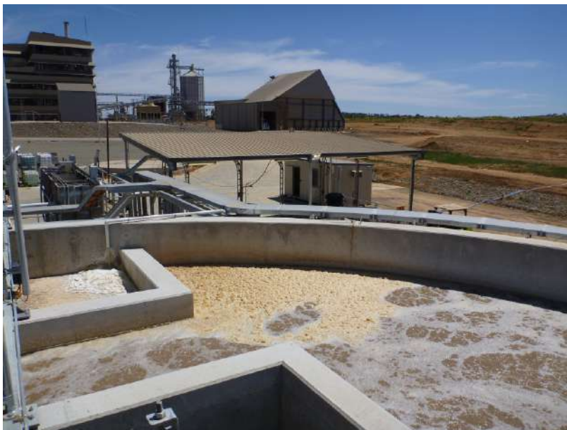
Figure 21 Aeration tank in the wastewater treatment plant
