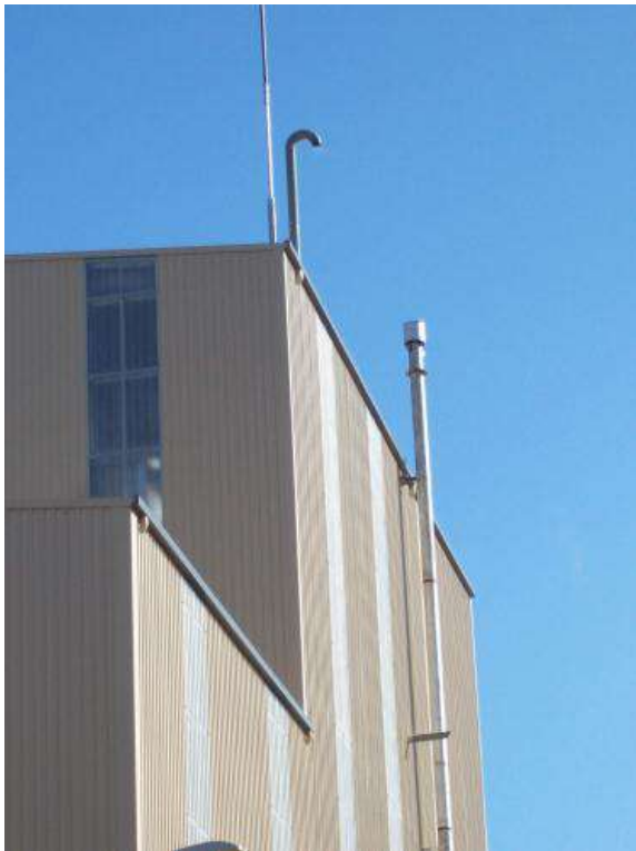
Figure 15 Refinery - filter blowing discharge point (left), steam boiler (right)
