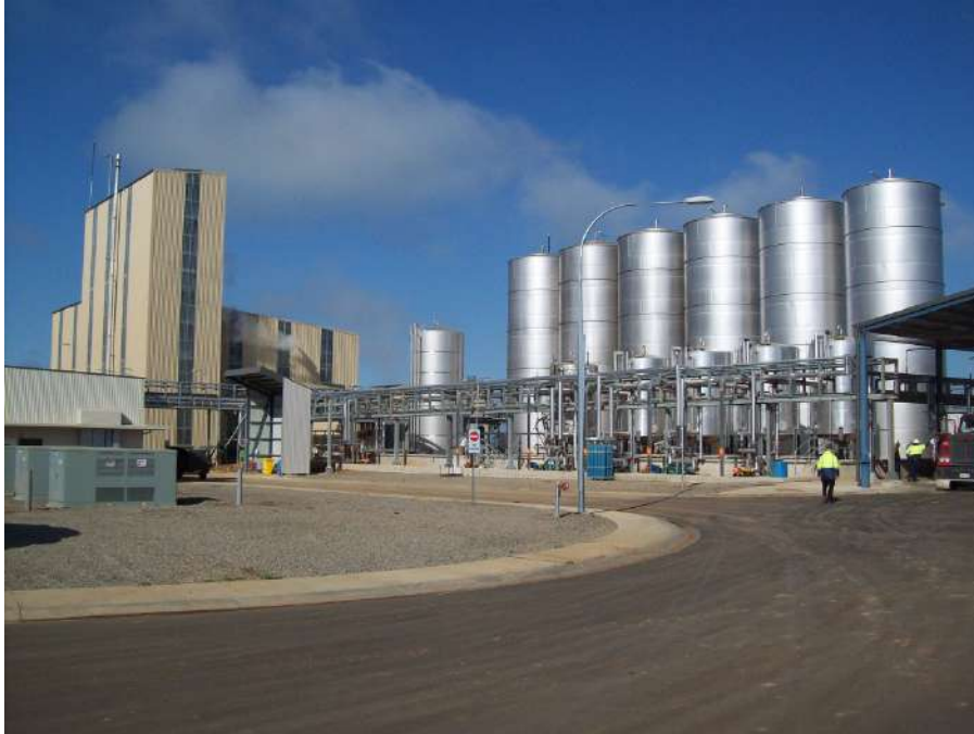
Figure 24 Crude and refined oil storage / tank farm
