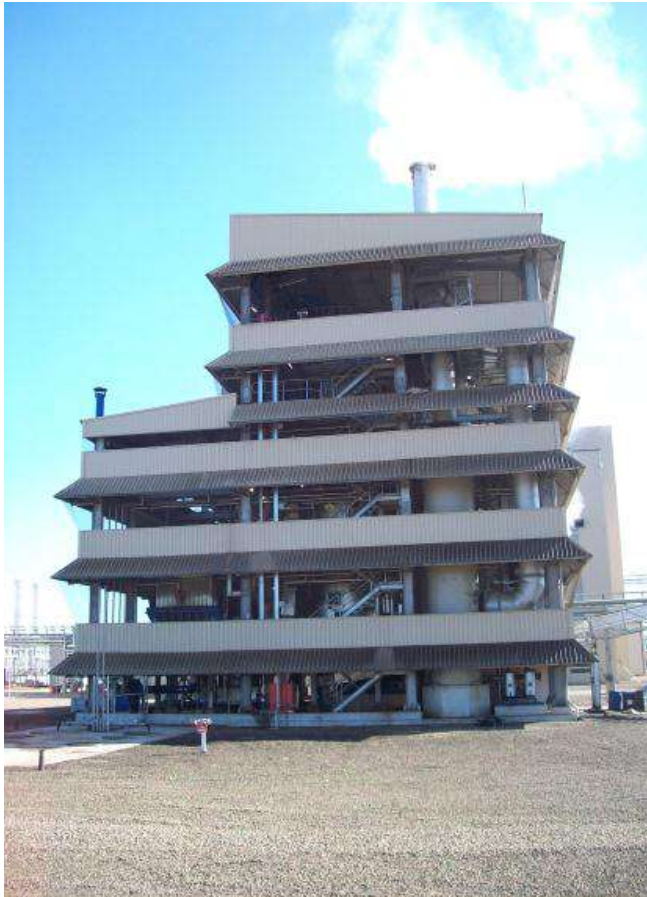
Figure 14 Solvent Extraction Plant – combined vent and scrubber (at right)
