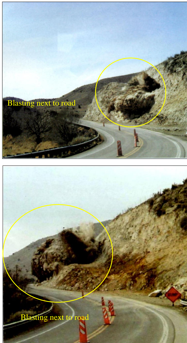
Figure 3 – Blasting next to Road (after Achuff and Aimone-Martin, 2005)
