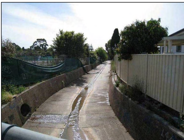
Photo 3: Stormwater culvert
