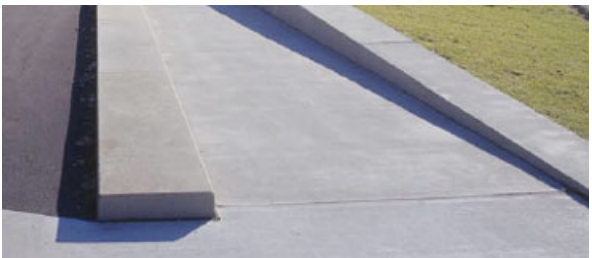
Cast insitu honed concrete footpaths
