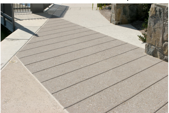
Exposed aggregate concrete paving
