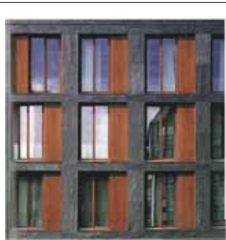
masonry facade panels and coloured inlaid glazing panels
