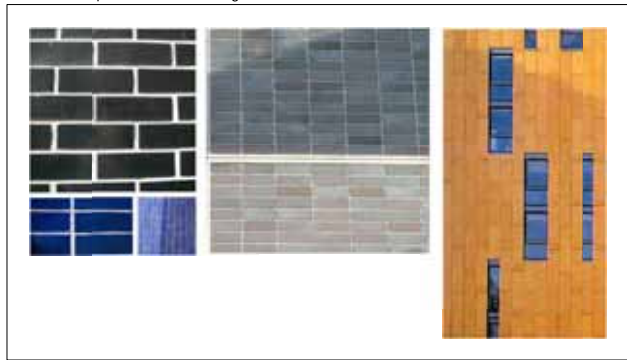
face brick panels and coloured glazed bricks
