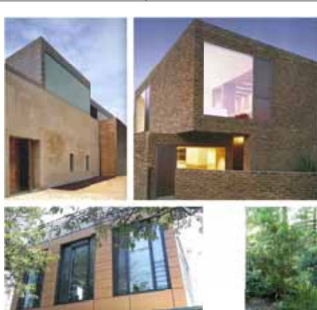
face brick and rendered masonry walls to Sinclair st.
