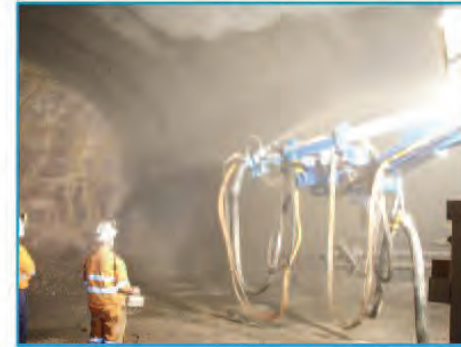
Additional roof support - shotcrete
