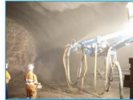
Additional roof support - shotcrete
