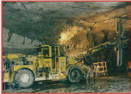
Installing rock bolts to provide roof support
